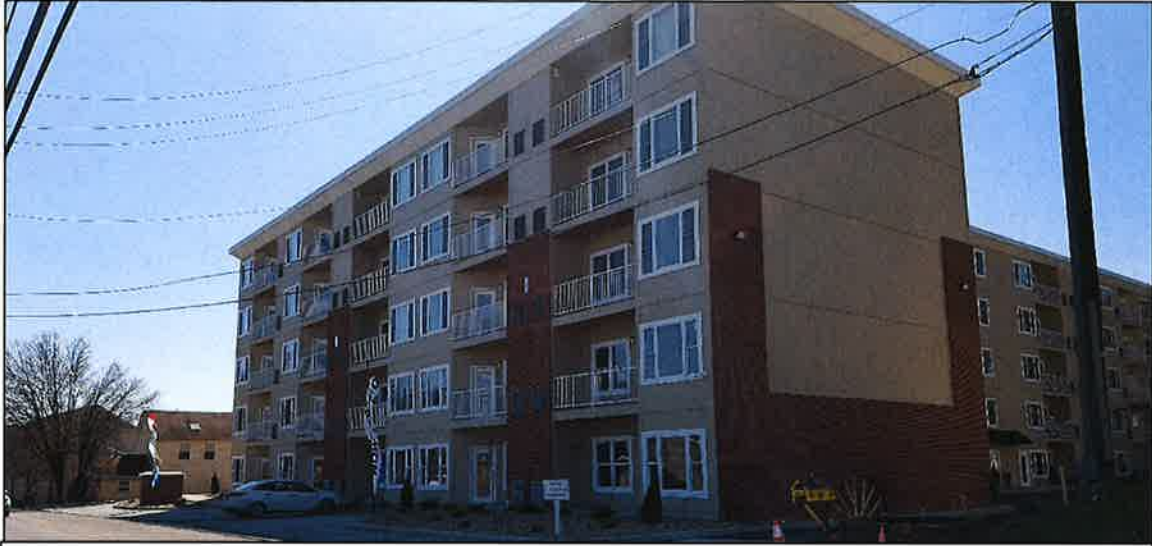
Constructed five story multifamily building approved through a Land Use Permit on 7-6-16
